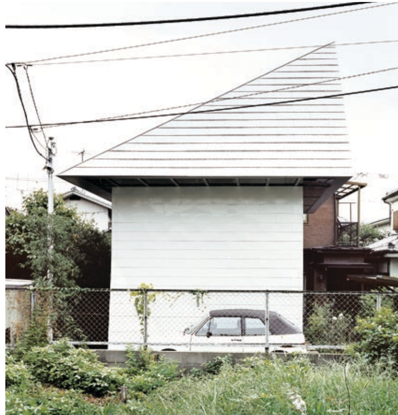
Kuća Gae, Tokyo, Japan, 2003. ▶ Gae House, Tokyo, Japan, 2003 ▶
